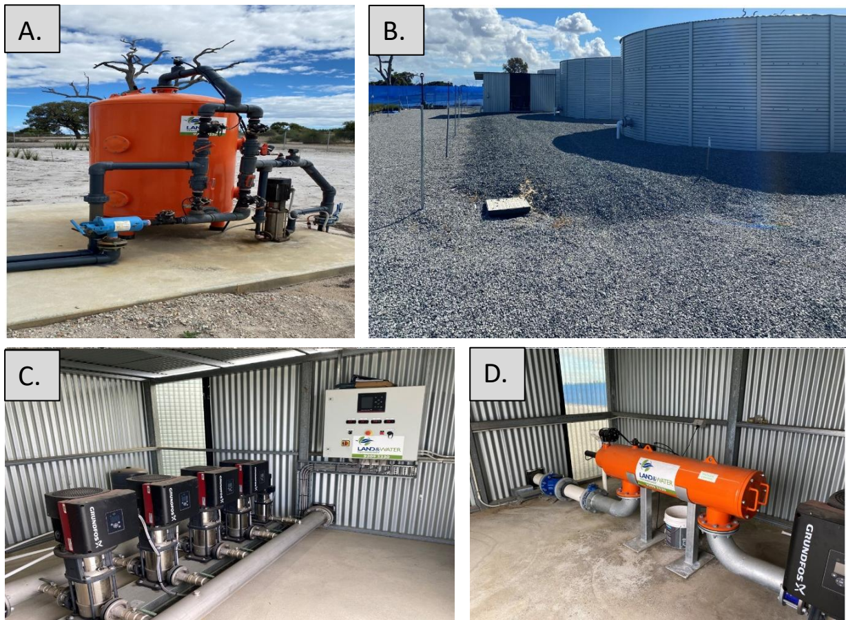
Figure 3. The new nursery has superior water quality thanks to the installation of modern A) Bore water filter. B) Large water storage facilities. C) Irrigation pumps with digital control and D) Screen filter.
