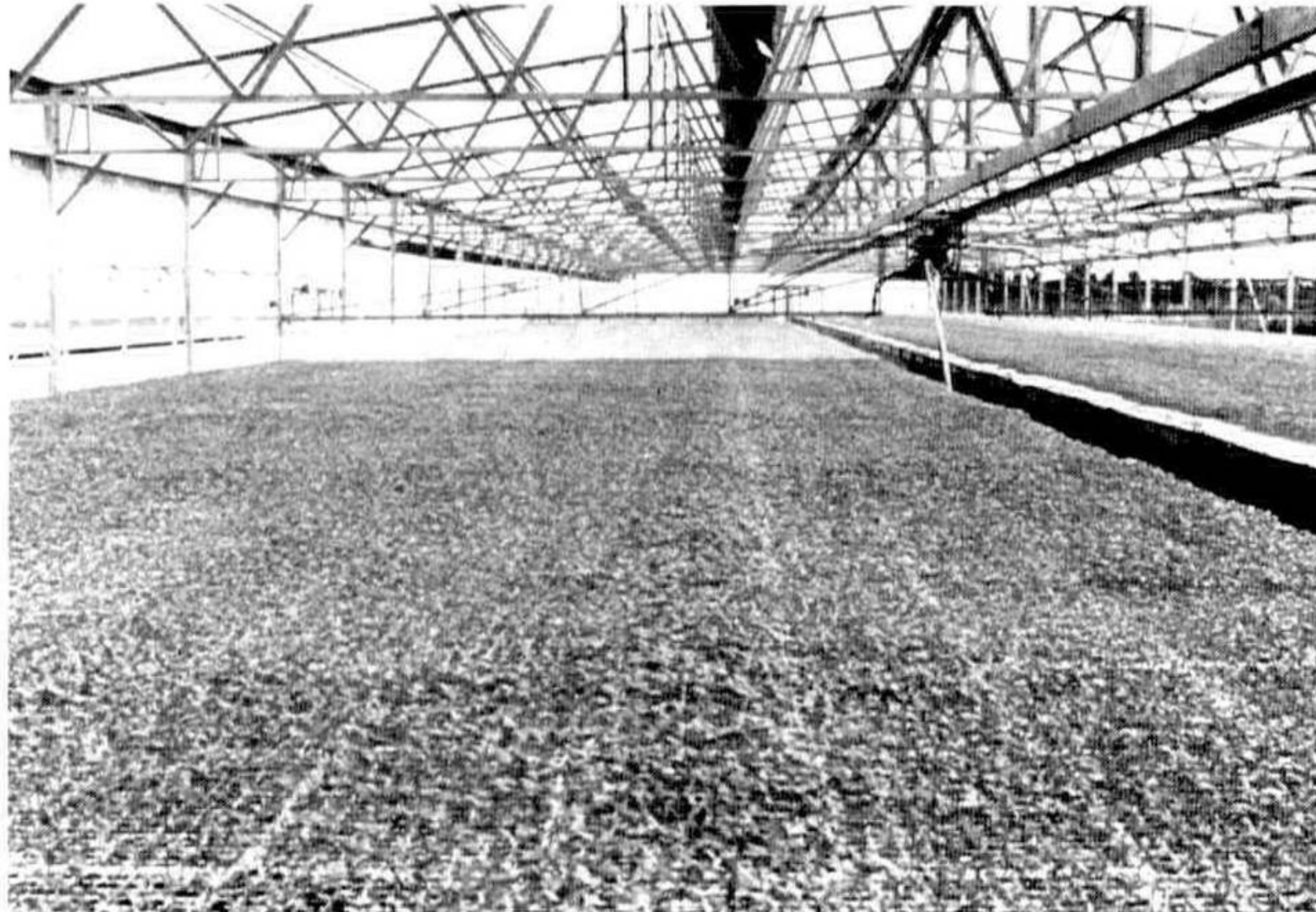
Figure 2. The Speedling greenhouse. Note the watering mechanism and side ventilation.
