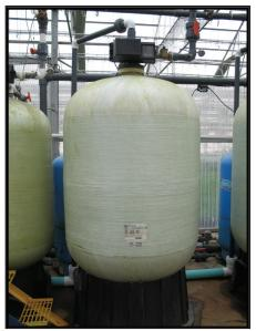
Figure 1. This reverse osmosis system was installed at a young plant production greenhouse to remove pathogens from water used to irrigate young plants.
