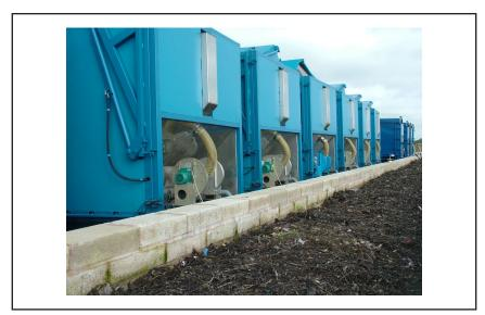
**Figure 3.** Composting in vessels destroys weeds/seeds and diseases (biofilter bed in foreground "scrubs" the vapour as it leaves the vessel). The green compost is then matured indoors with further aeration and temperature monitoring, then screened prior to further maturation and testing before blending.
