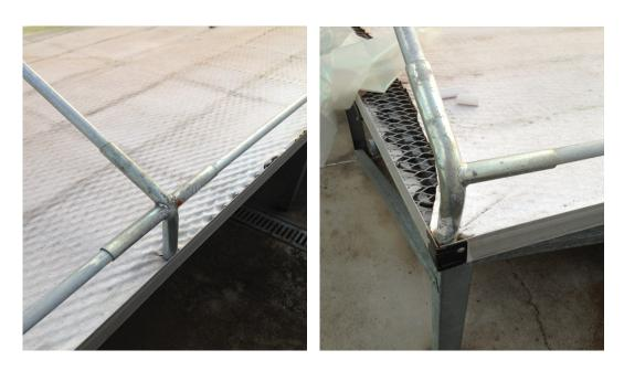
Fig. 2. Conduit electrical metallic tubing connectors used for the construction of the plastic tent.
