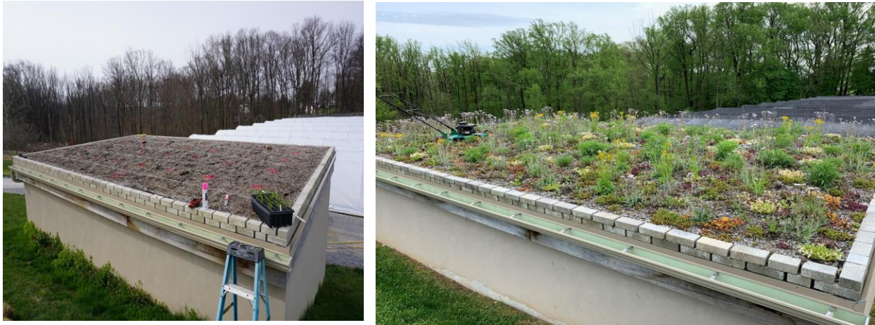
Figure 4. Establishing a green roof in Landenberg, Pennsylvania.
